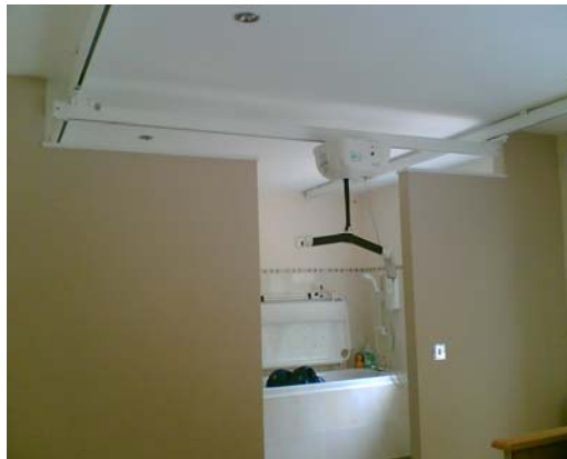
Typical example of a 2-Room Covering H-System
